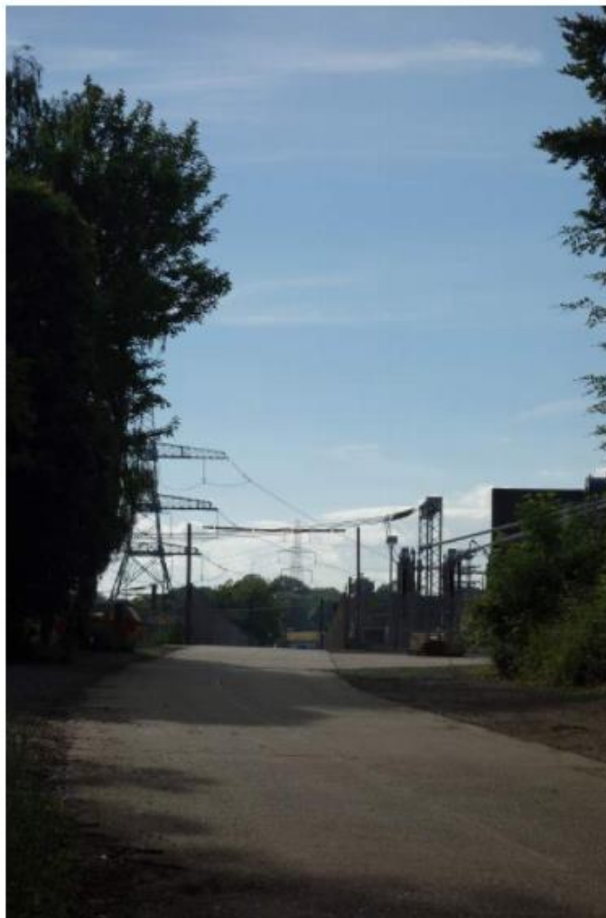
The current substation site in Lovedean – the Aquind Interconnector's converter station will be located close to this site.
